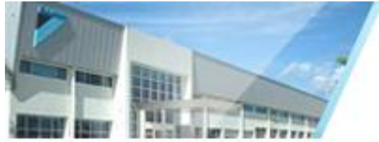
Daikin Compressor Industries Ltd.
